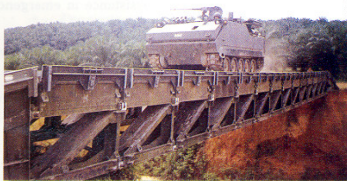
Providing fixed bridge (MGB) under Mobility Task
